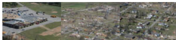
Damage at Marmaduke, Arkansas
