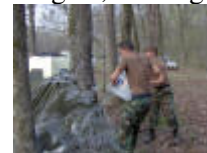
Cadets from the 99th test shelter for waterproofing
